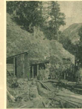
TUNNEL AT NOBLE MINE
