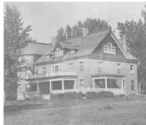
The beautiful home built by Winthrop Raymond. (Was destroyed by fire.)
